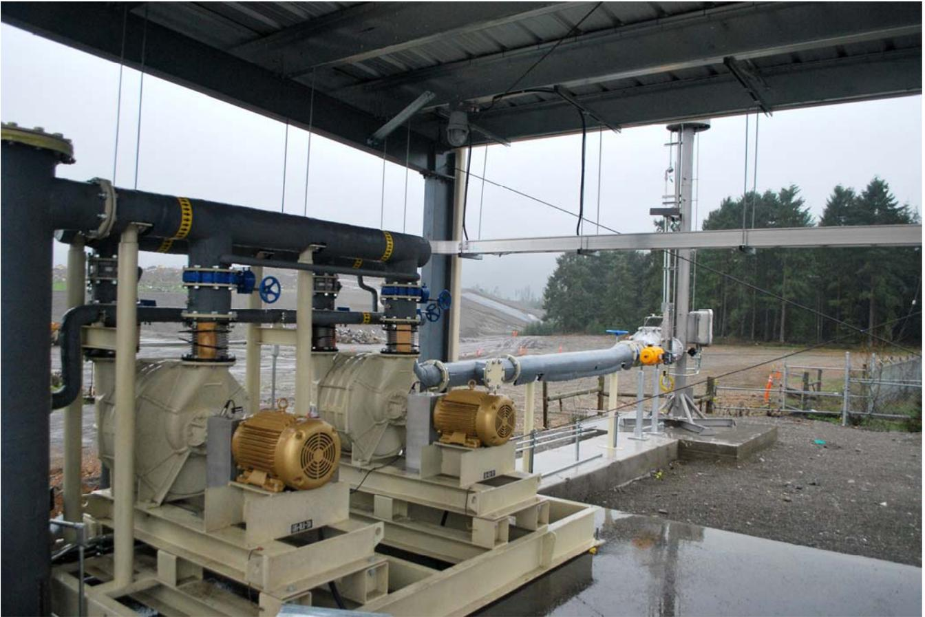
*Picture of the blowers that are connected to the gas flare and overhead structure that was built to protect the equipment – conforming to the strict electrical requirements around gas equipment.*
