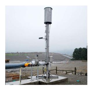
Picture of the new landfill gas flare was recently installed; thermocouples and infrared sensors will monitor the flame to ensure proper operation. There are pneumatic shut off valves and a flame arrestor also in place for added safety. The gas flare is scheduled to be in operation by mid-January, 2016.
